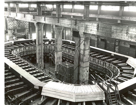
Manhattan project Calutrons that enriched uranium via electromagnetic separation – no longer operating
