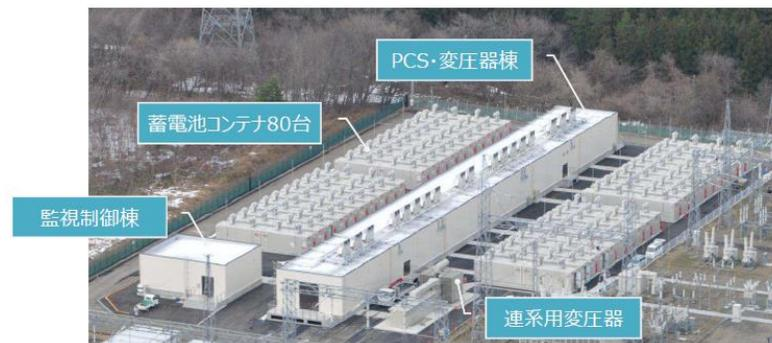
Figure 2: Lithium batteries at Tohoku Electric Power Company's Nishi-Sendai substation
