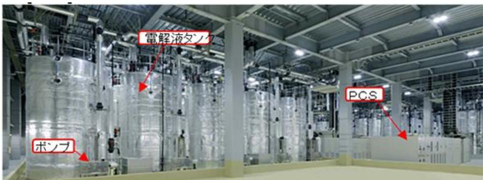
Figure 1: Redox flow battery at the Minamihayarai substation of Hokkaido Electric Power Co.
