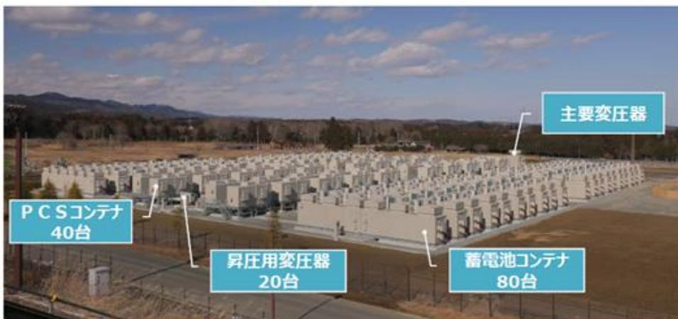
Figure 3: Lithium batteries at Tohoku Electric Power Company's Minamisoma substation
