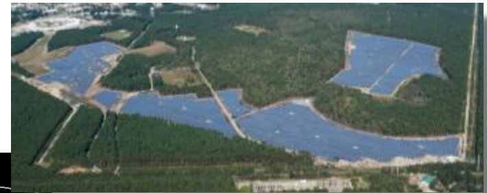
Long Island Solar Farm
