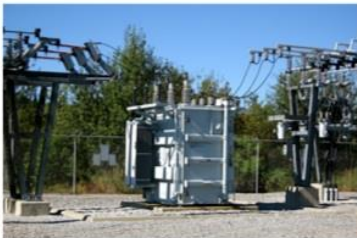
8000 lbs, 60 Hz Distribution Transformer
