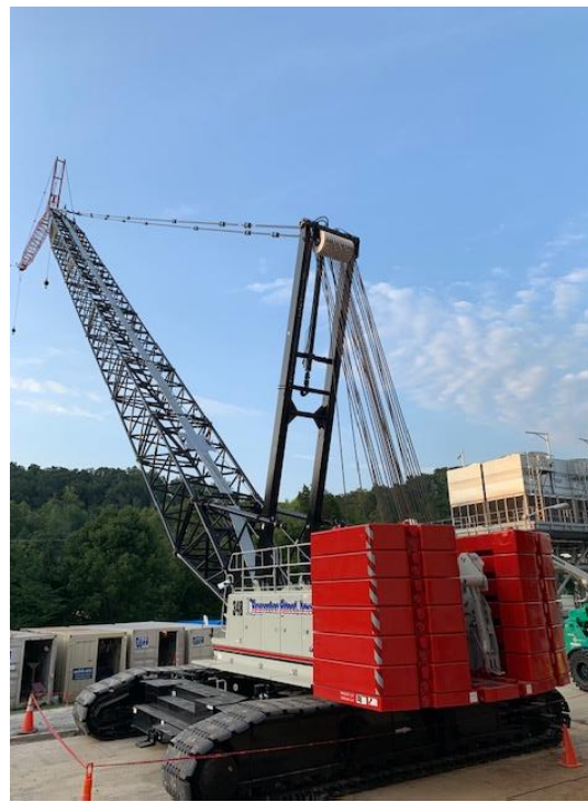
Crane to lift cooling towers to the roof
