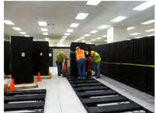
Hopper installation, August 2010
