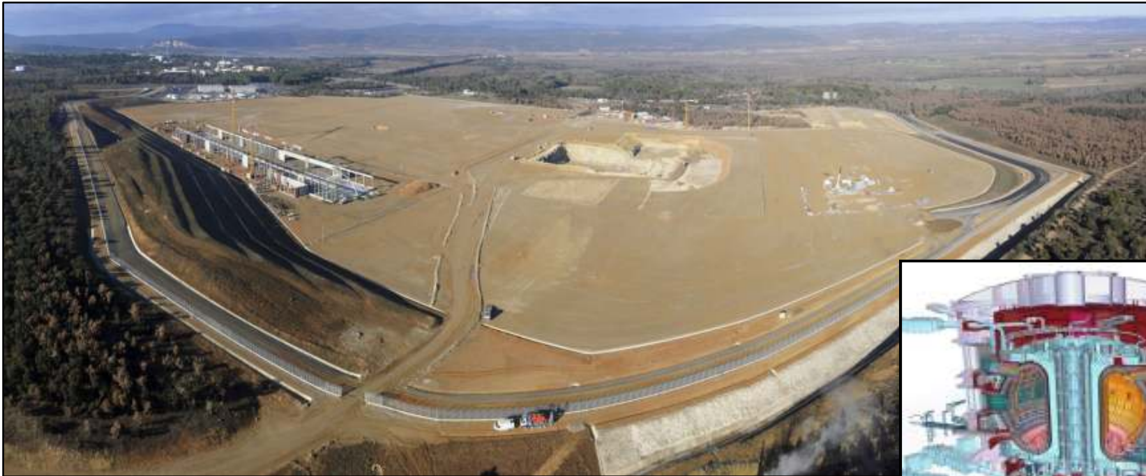
Site construction is underway in Cadarache, France
