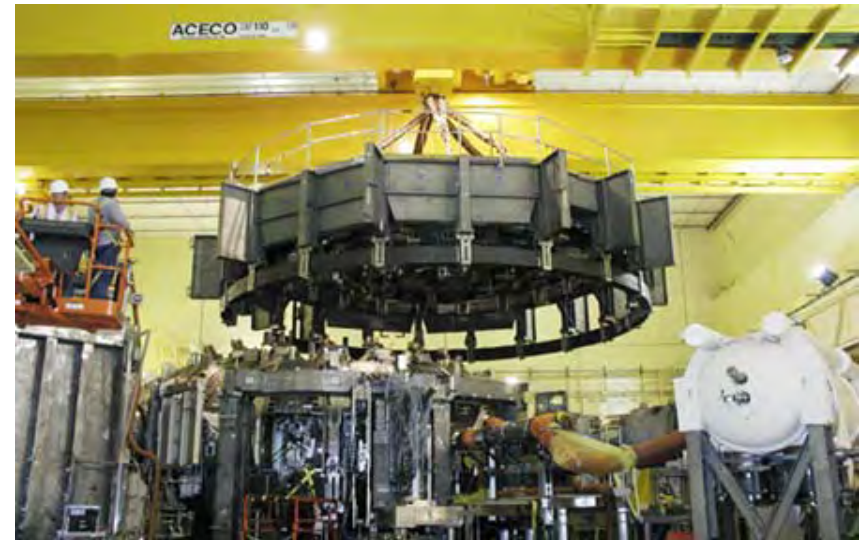
Removal of the TFTR Umbrella Structure
