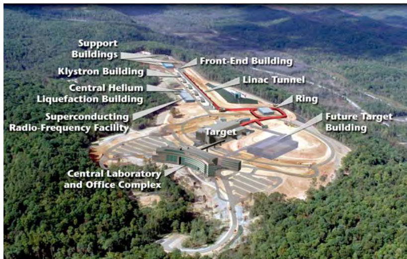
Artist's Conception of the Finished Facility Overlaid on the October 2000 Aerial View
