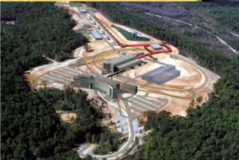
Site plan of the Spallation Neutron Source being built at Oak Ridge National Laboratory in collaboration with ANL, BNL, LBNL, and LANL
