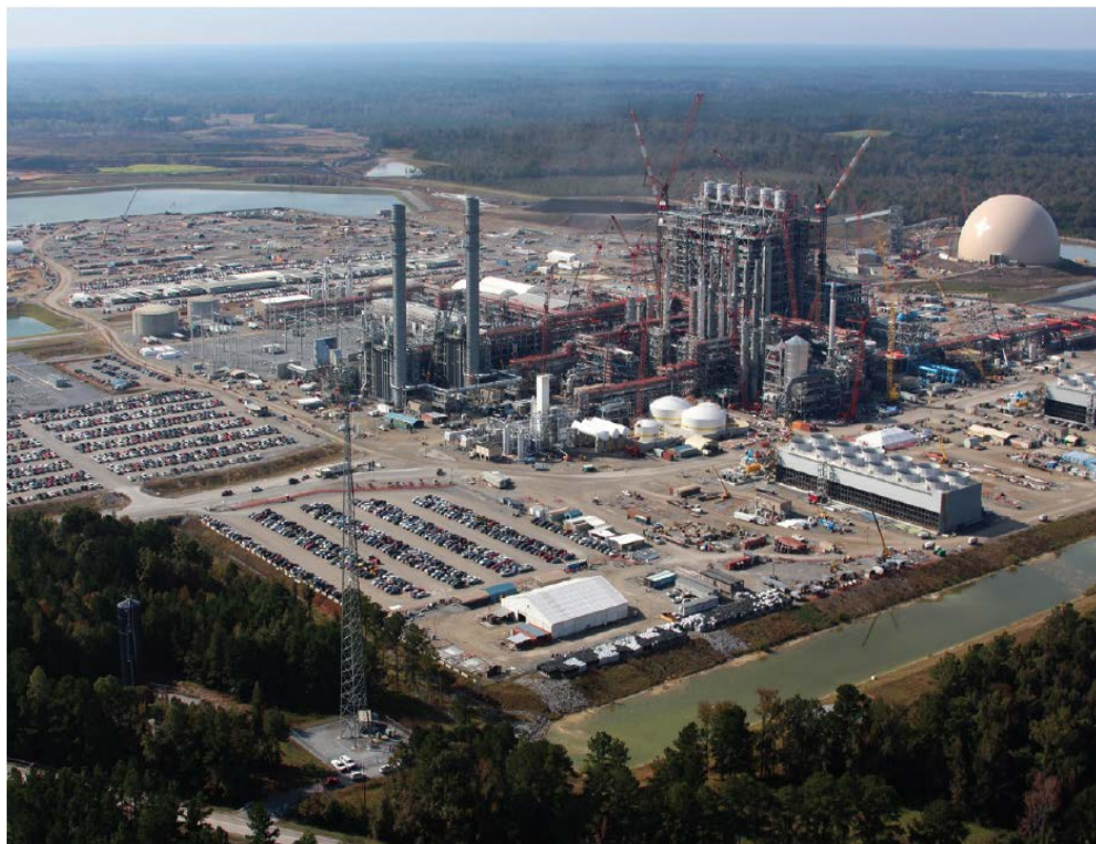
Southern Company Kemper Project, IGCC + CC + EOR Credit: Mississippi Power
