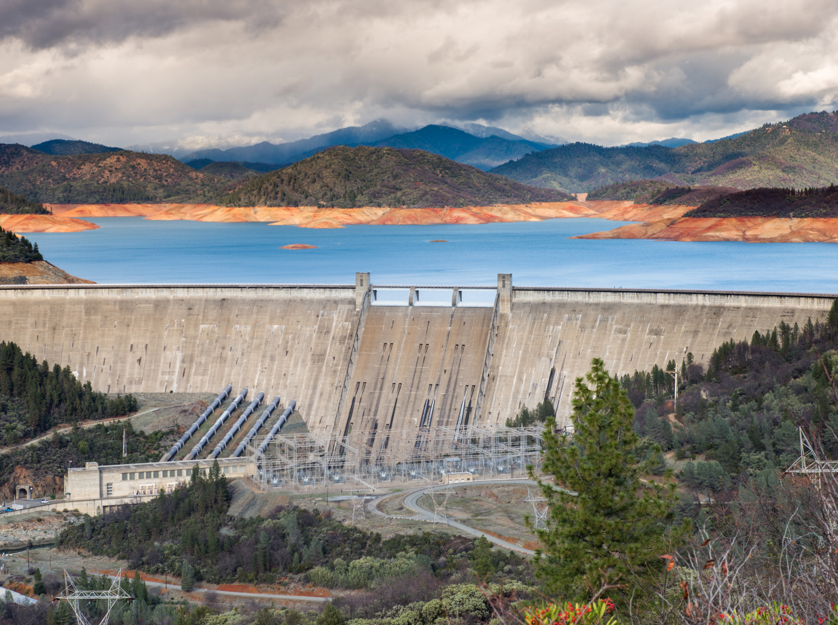
Shasta Dam, Calif. Courtesy Adobe Stock
