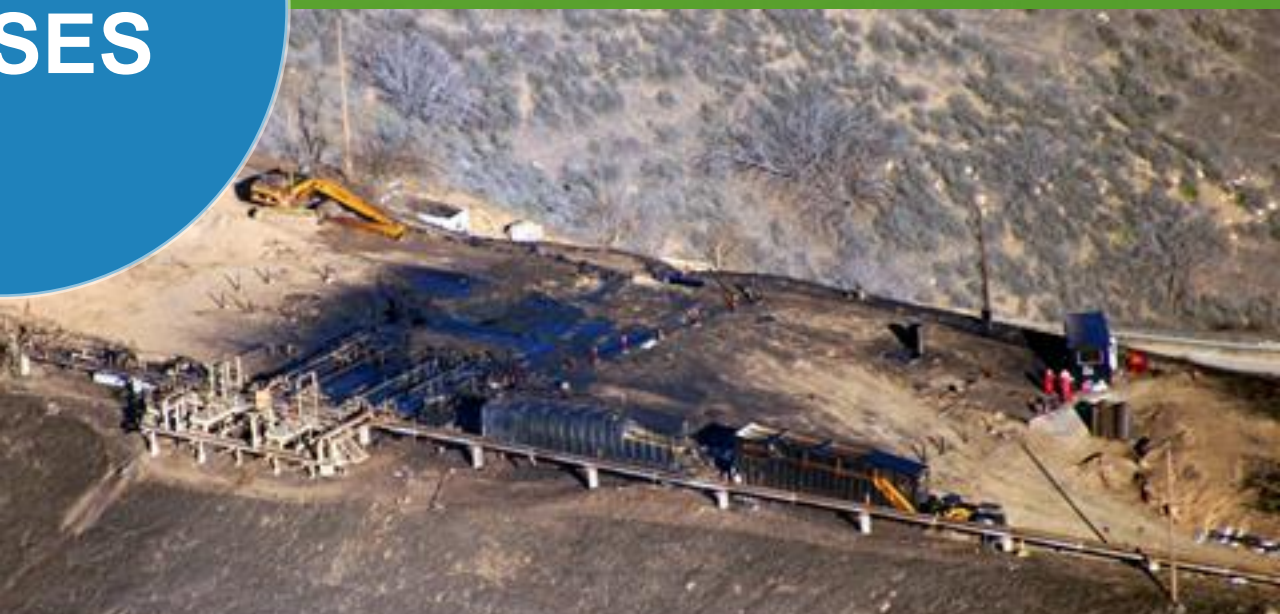
Aliso Canyon Gas Leak
