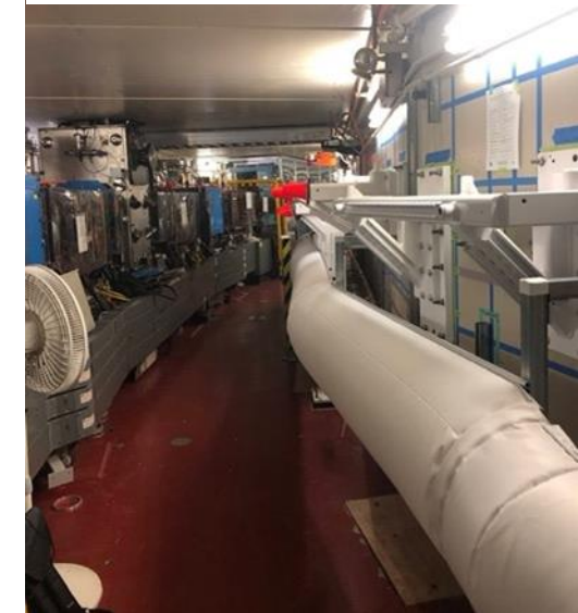
ALS-U accumulator ring supports
