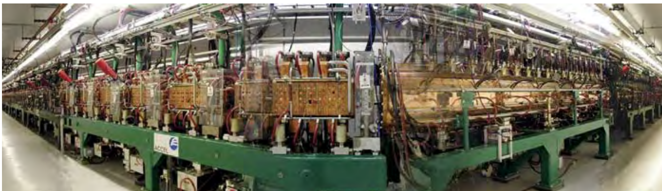
Five national laboratories collaborated to build the Spallation Neutron Source at Oak Ridge National Laboratory. Photo courtesy of Oak Ridge National Laboratory
