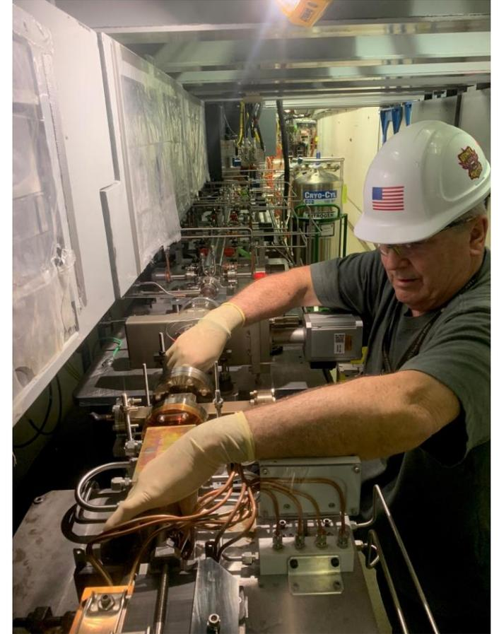
Installation of the kicker absorber in APS Sector 39, the **final** component of the MBA storage ring, completing installation.
