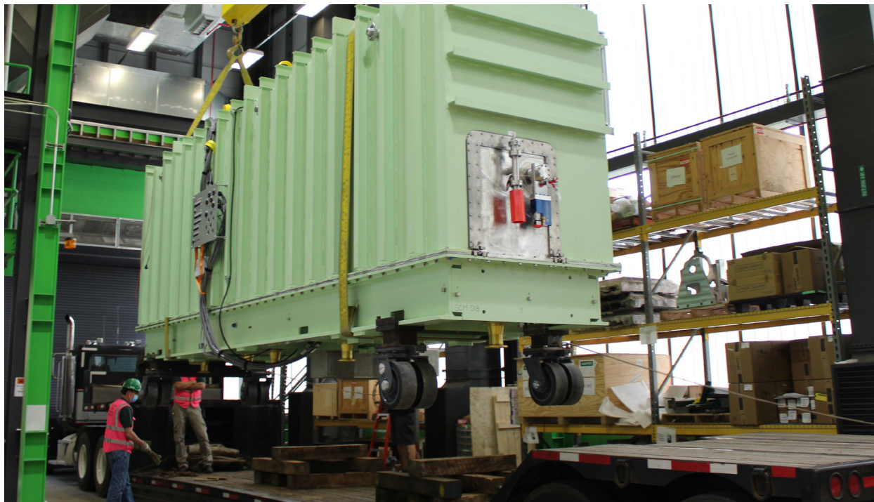
Fig. 3.2. Facility Construction Continues During the Pandemic. Workers at the Facility for Rare Isotope Beams (FRIB) at Michigan State University move a cryomodule into the linear accelerator (linac) tunnel. As the start of user operations in early 2022 nears, the FRIB team commissioned the entire linac, including all 46 cryomodules, in April 2021. The commissioning team was distributed to five separate control rooms to comply with COVID-19 workplace safeguards. [Courtesy Michigan State University]
