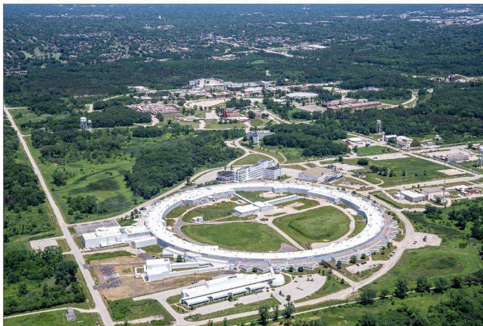
Figure 5.2.1: Aerial view of the APS
