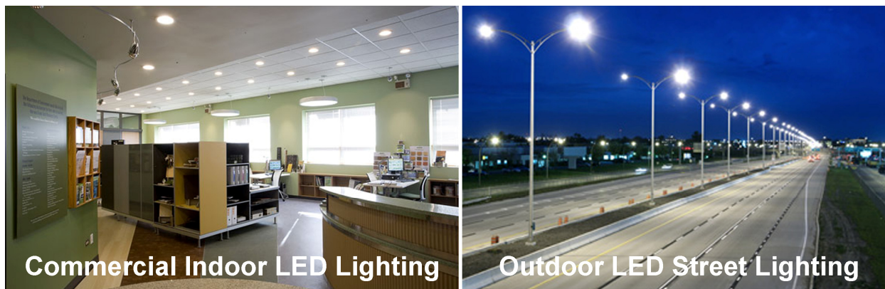
Figure 8-3 (Left) The Chicago Center for Green Technology uses indoor LED lighting to reduce its energy demand for lighting by 64%, freeing the building’s solar panels to produce electricity for other uses. Source: Eric Taub, New York Times, 2/29/2009. (Right) With superior color quality and lifetime and high lumen output, LEDs are the emerging technology for the next generation of outdoor lighting. Source: Luminus Devices, Inc.
