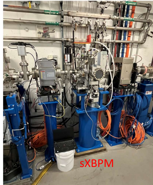
sXBPM installed in 23-ID FOE
