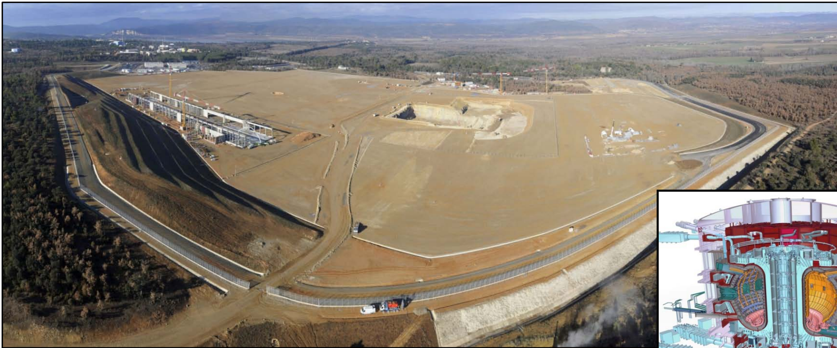
Site construction is underway in Cadarache, France
