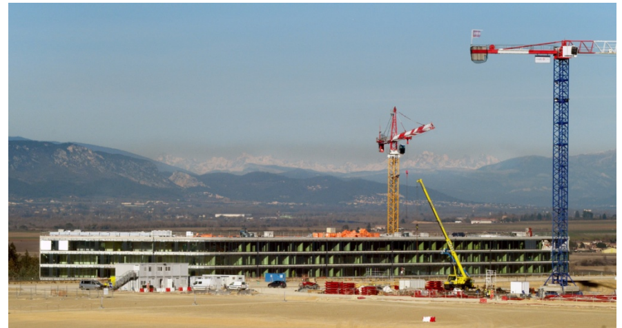
ITER Headquarters Bldg
