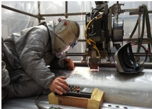
Inner shell welding
