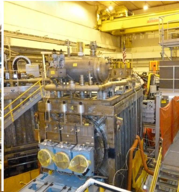
Beam Box being populated with components
