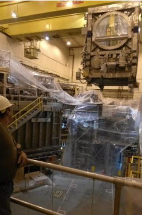
Beam Box being lifted over NSTX
