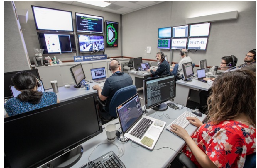
Remote Control Rooms Enable Remote Collaboration in Experiments and Operations
