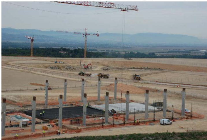
The concrete foundation for the Poloidal Field Coil Winding Facility is being put in place
