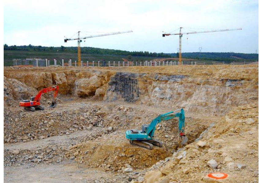
Excavation of the Tokamak Building
