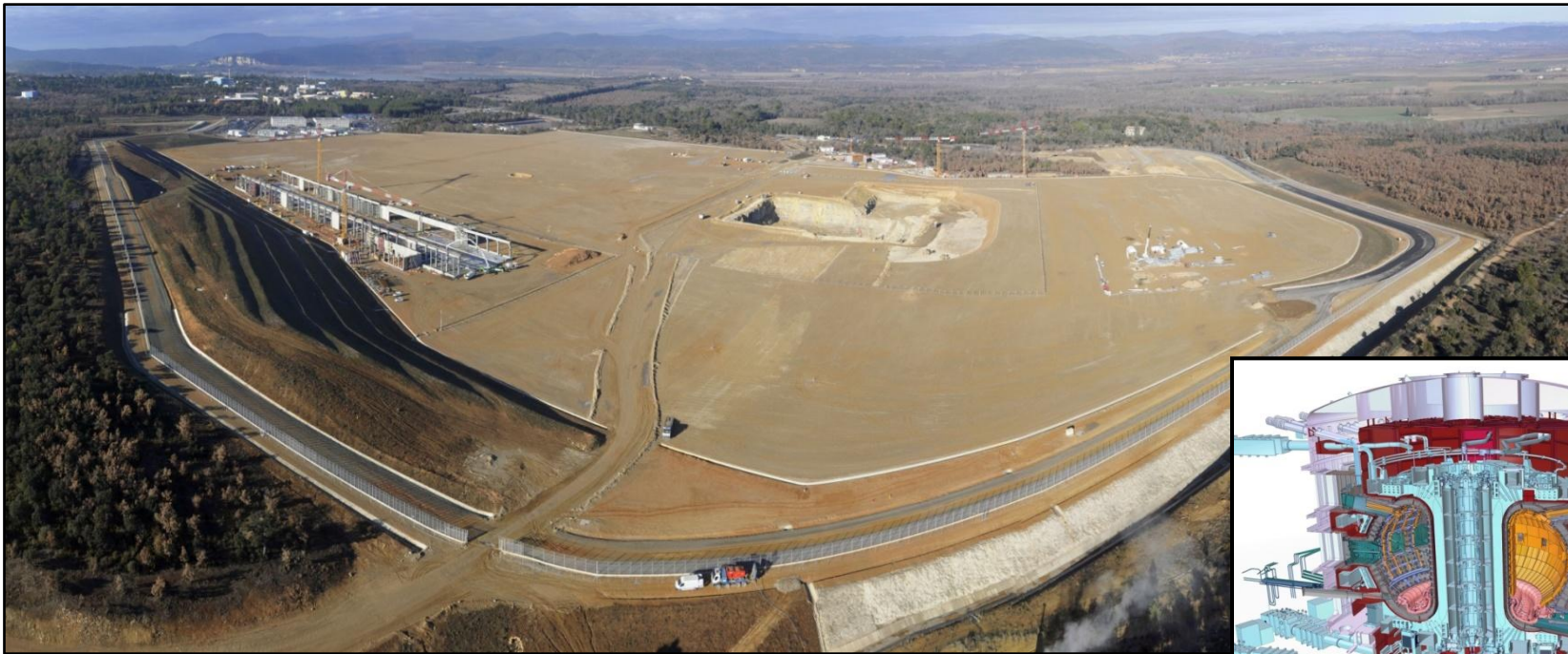
Site construction is underway in Cadarache, France
