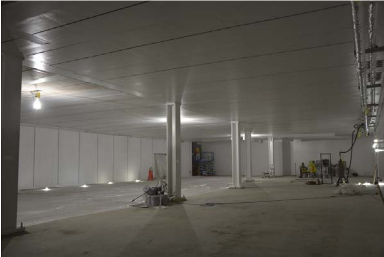
Tunnel warm and painted
