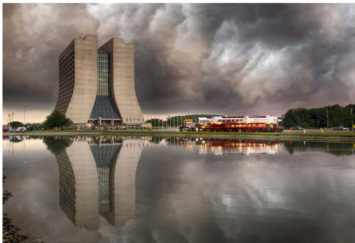
Superconducting coils transported from Brookhaven arriving at Fermilab 5200 Amps
