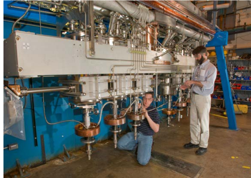
Cavity string suspended from the lid, ready to be dropped into the vacuum vessel.
