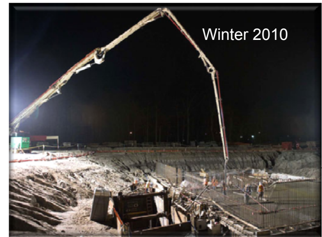
Pouring the foundation for the Hall D complex.
