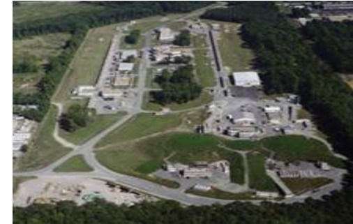
Continuous Electron Beam Accelerator Facility (CEBAF) Jefferson Lab, Newport News, VA
