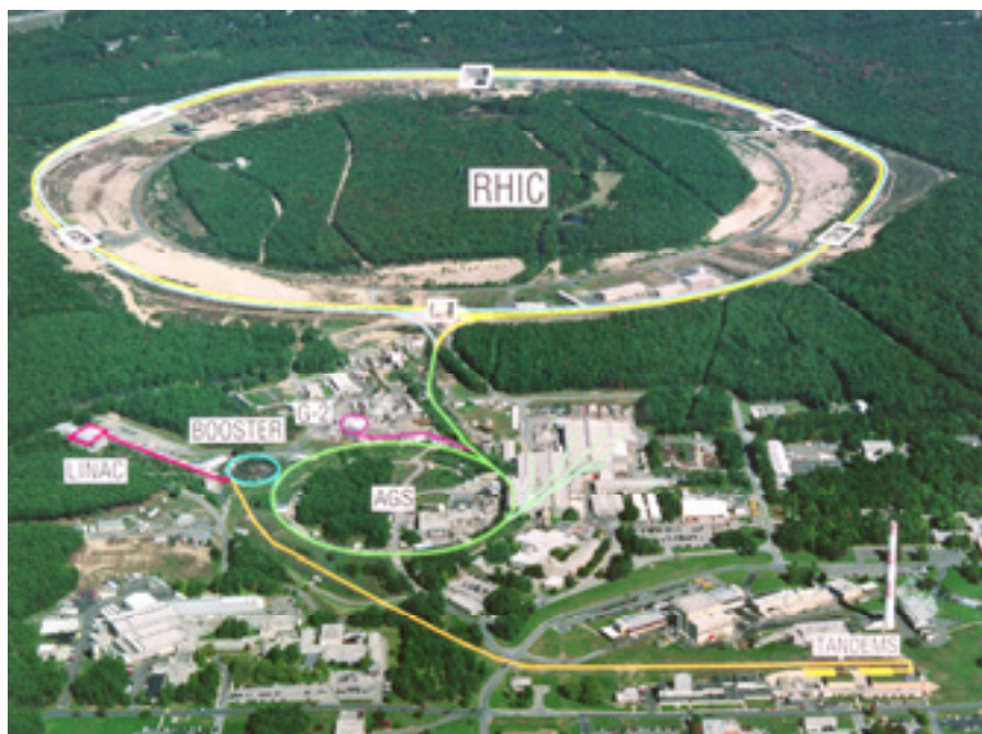
Figure 1. The Relativistic Heavy Ion Collider complex at Brookhaven National Laboratory in New York. The complex is comprised of several accelerator facilities joined together to provide beams that are brought into collision in detectors located along the Relativistic Heavy Ion Collider ring. Image courtesy of Brookhaven National Laboratory.
