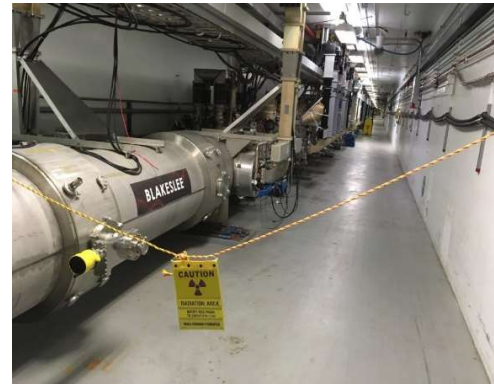
hazards due to activation
