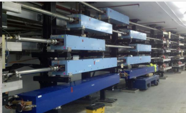
~500 Large Dipoles powered by >40 HVPS
