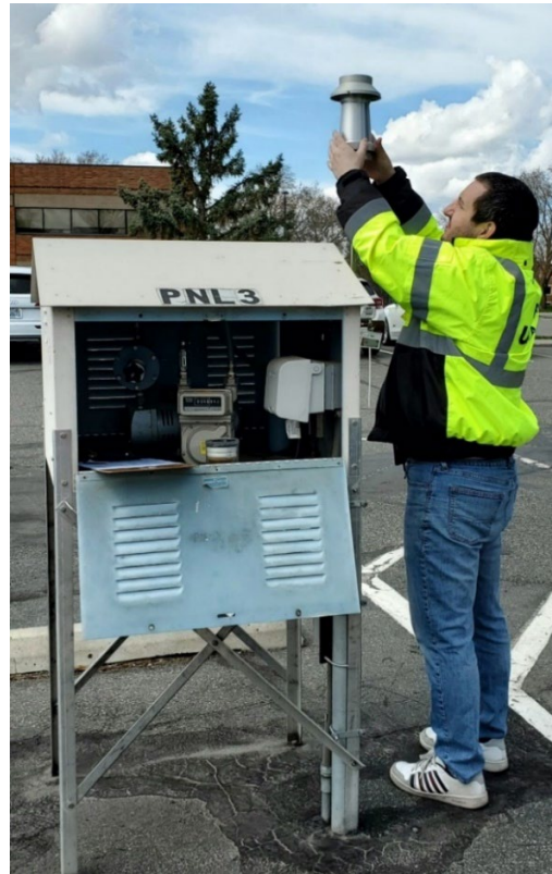
Staff Member Maintaining an Air Sampling Station
