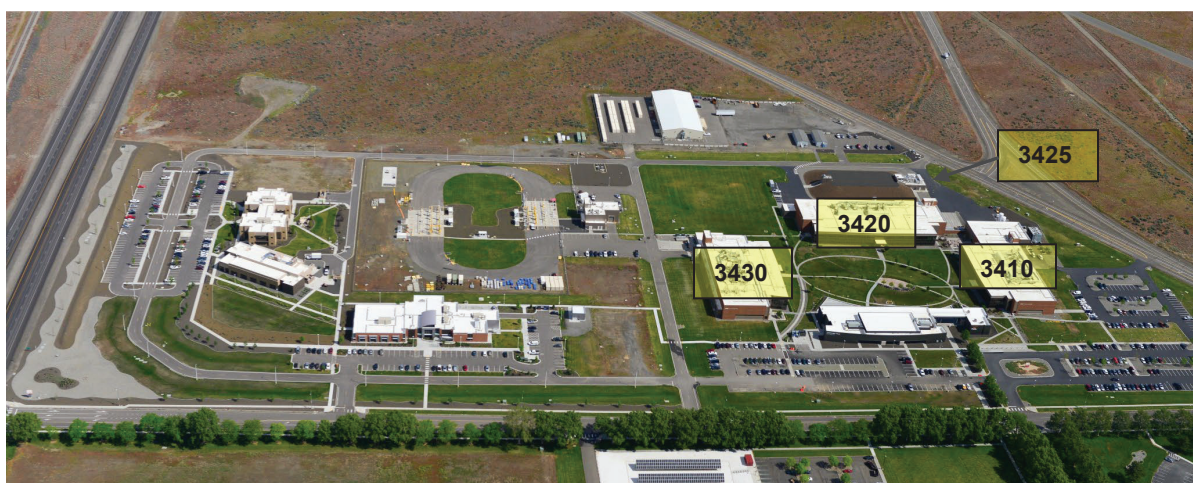
Figure 1.3. PNNL-Richland Campus Physical Sciences Facility (PSF) with Buildings Identified
