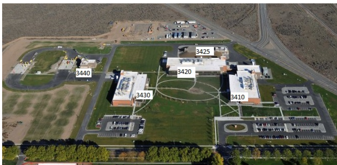
Figure 1.3. PNNL Campus Physical Sciences Facility (PSF) with Buildings Identified
