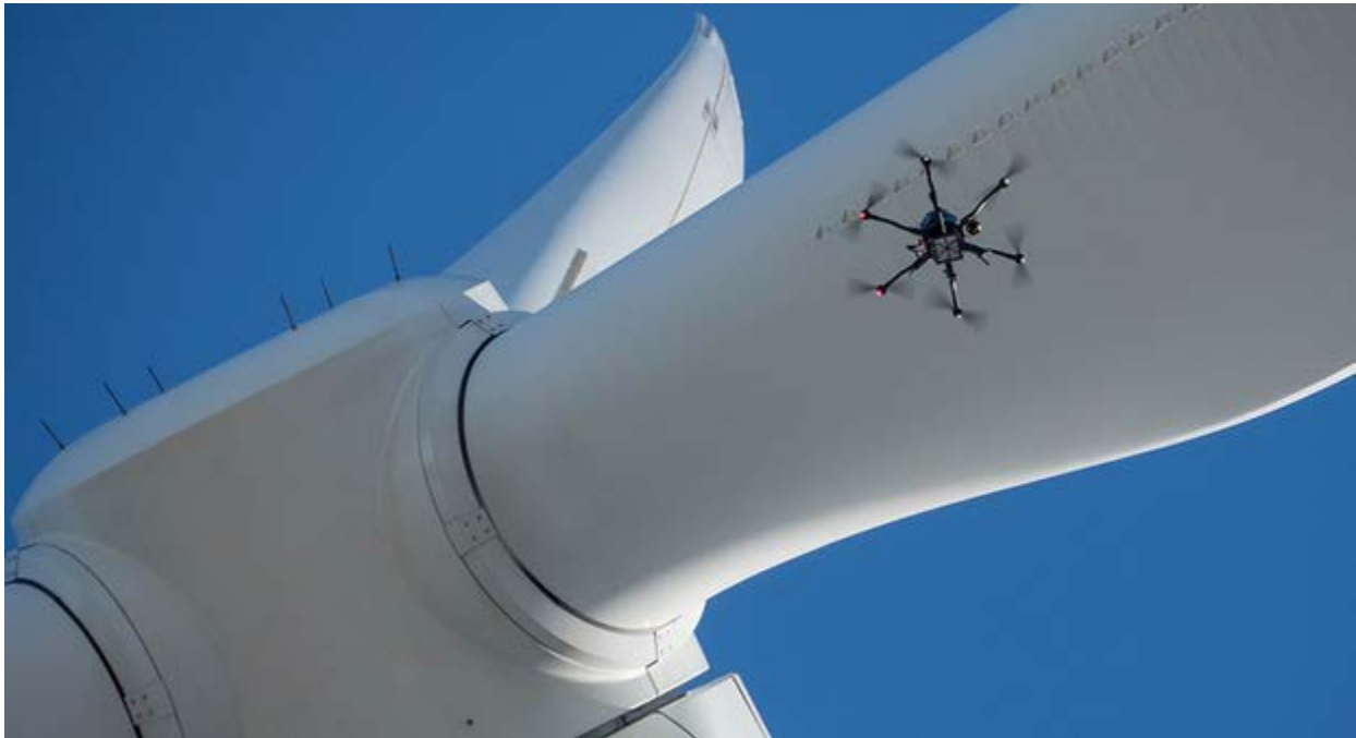
Figure 16: SkySpecs Drone Inspecting a Turbine
