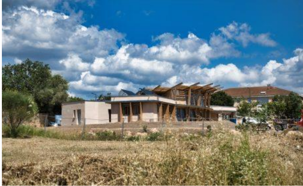
Figure 14: DualSun Hybrid Panels on Restaurant in Marseille Source: DualSun
