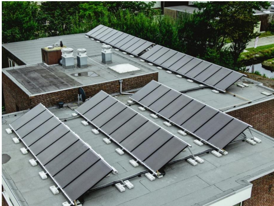
Figure 11: Abora Solar Installation at a Hotel in Ruigrok, Netherlands Source: Abora Solar
