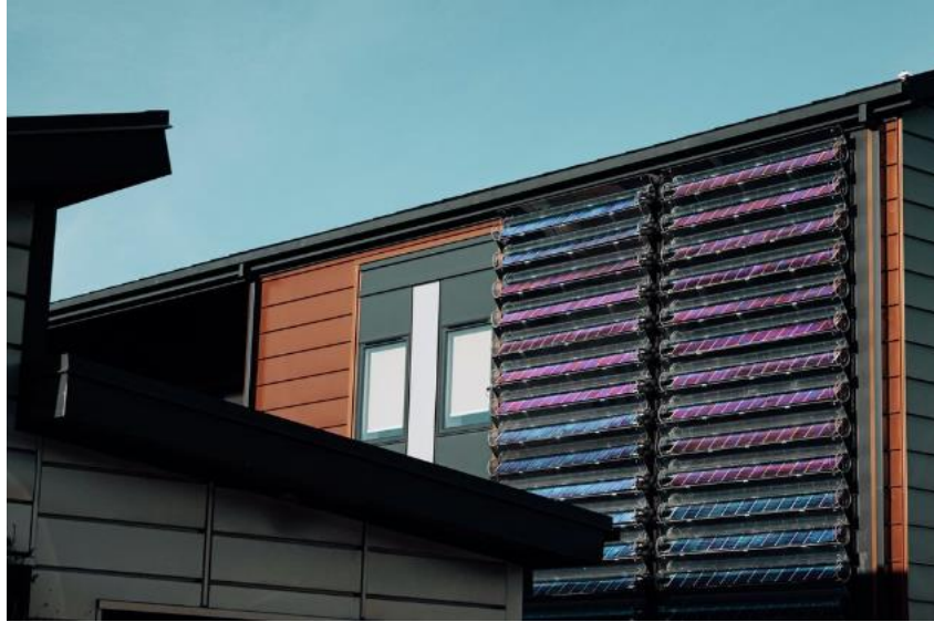
Figure 16: VirtuPVT Installed at SPECIFIC
