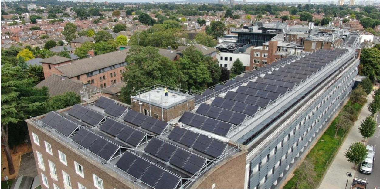
Figure 19: Triple Solar’s PVT System on The University of West London
