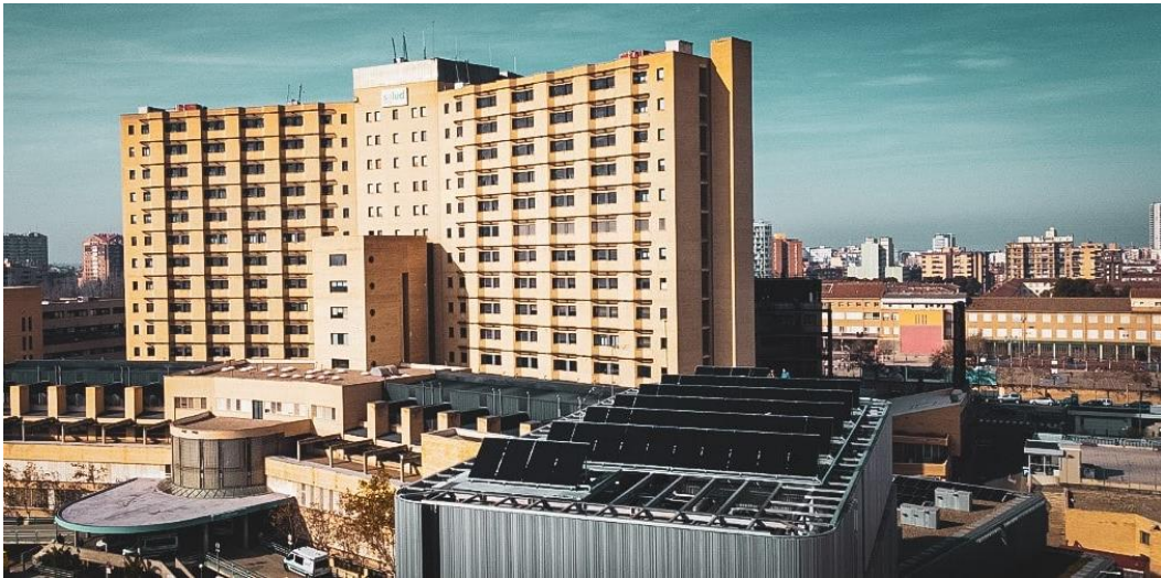
Figure 10: Abora Solar Installation at CIBA Biomedical Research Center in Spain Source: Abora Solar
