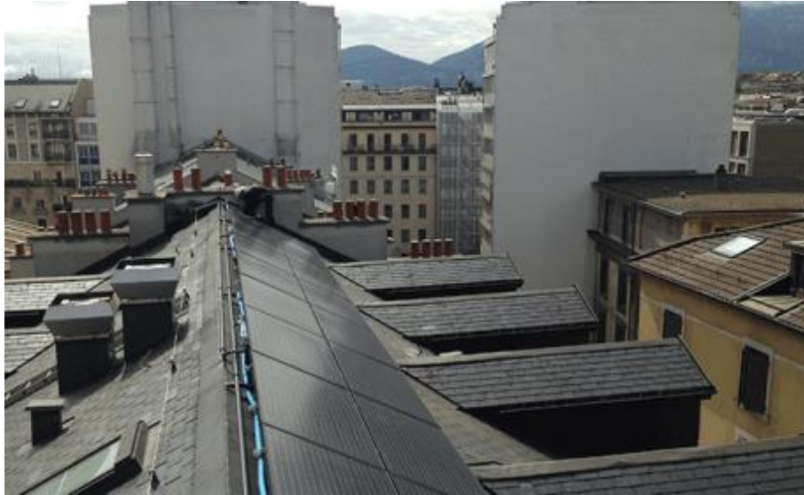
Figure 13: DualSun Hybrid Panels on Building in Switzerland
