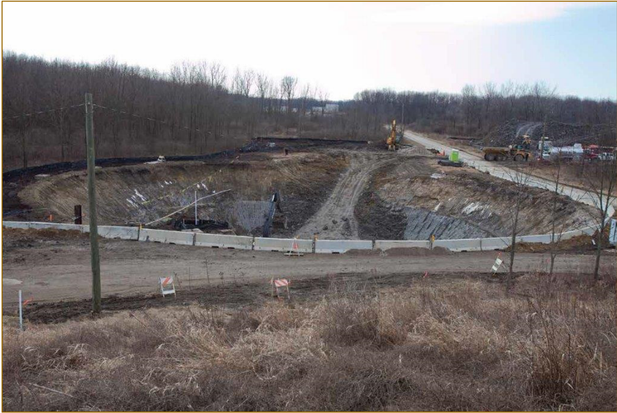
Figure 2.1-5 Previous Fermilab Excavation for LArTF Underground Experimental Hall
