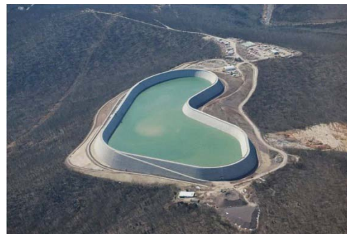
Pumped Hydro (Taum Sauk) 400 MW
