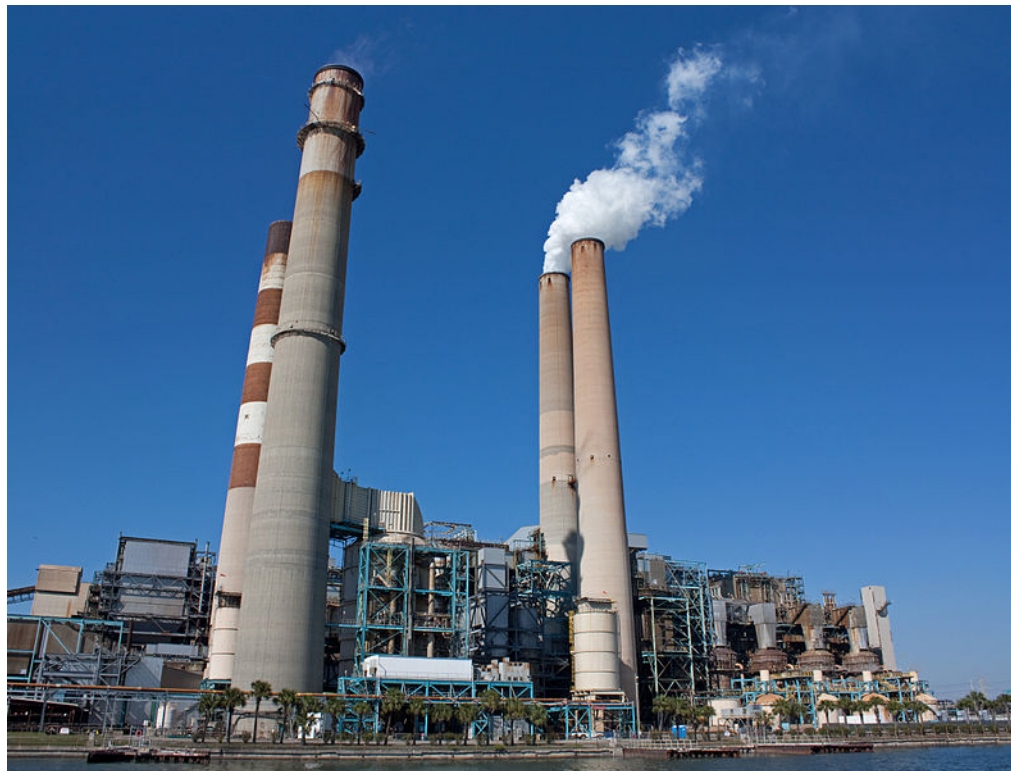
Big Bend Coal Power Station, Apollo Beach, FL
